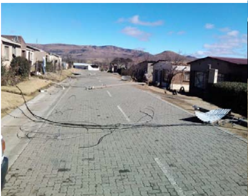
Tlholong Tornado debris
